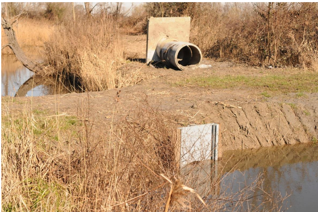
Fig. 9. Existing concrete sluice gate.
