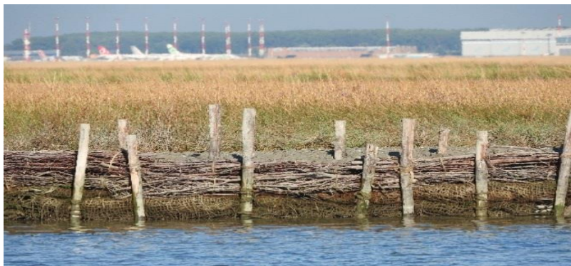
Fig. 17. Fascines side view protecting salt marsh edge in Venice Lagoon
