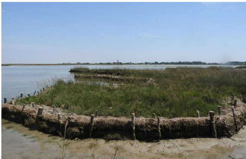
Fig. 18. Fascines in Venice Lagoon protecting salt marsh edge realized in LIFE VIMINE project
