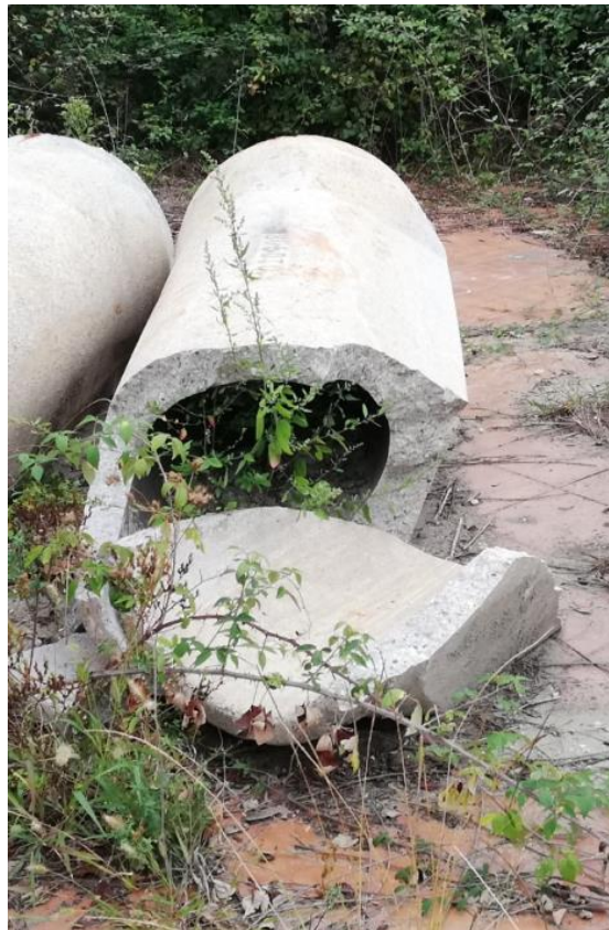
Fig. 12. Existing concrete pipe to be replaced
